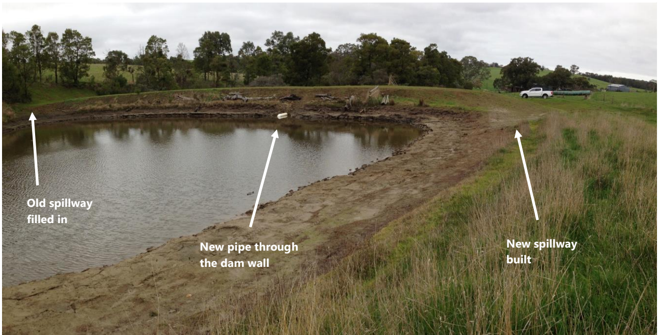
The Flaxley dam after works were completed
