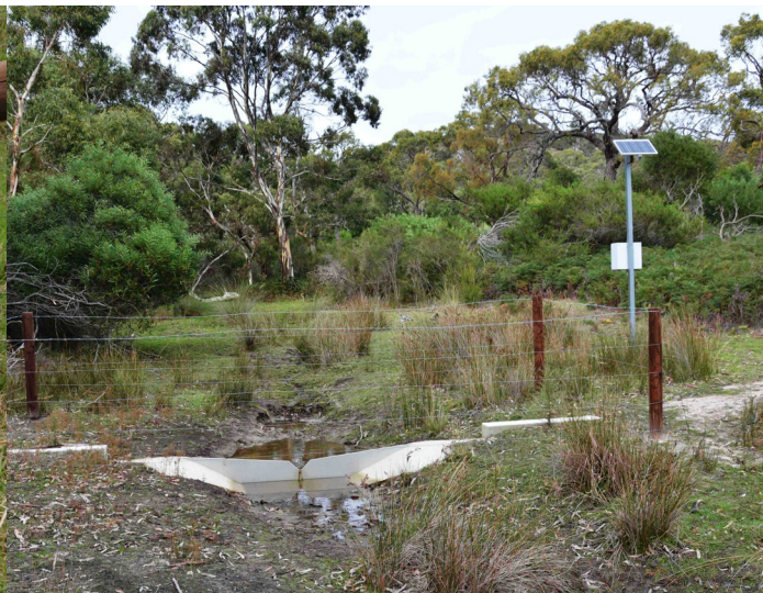
A sensor at a small weir above the dam measures in-flows.
