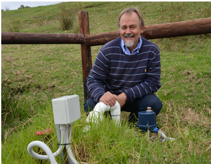
Peter Gale with the series of pipes, sensors and valves that comprise his property's method of passing low flows.
