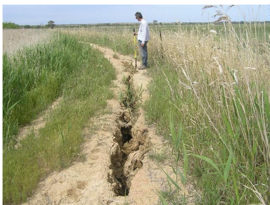
Figure 1: Soil cracking within a LMRIA levee bank
