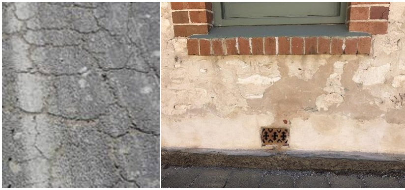
Figure 8 Salinity affected road and building foundation. Photo credit: NSW Government
