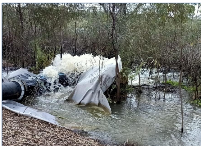
Figure 6. Pump outflow into temporary basin (T1)
