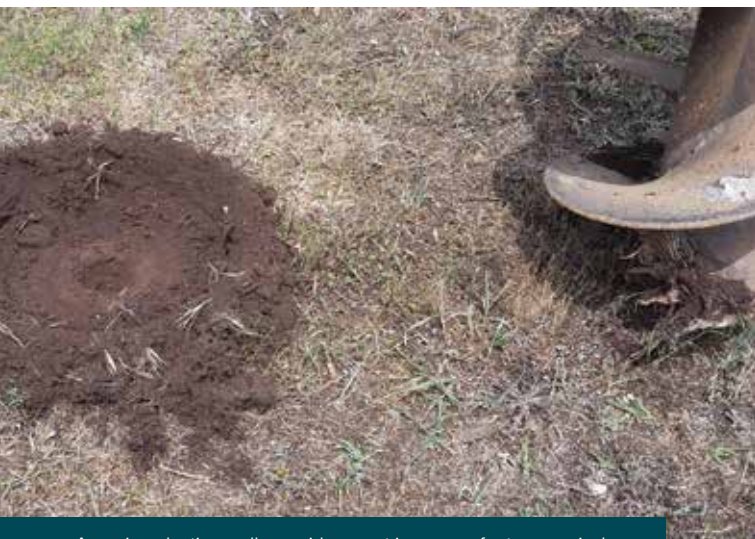
Augering planting wells provides great insurance for tree survival
