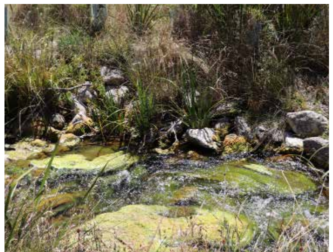
Image 8: Fish Passageway (this gentle gradient has been specifically designed to allow fish to swim upstream and access the ponds from the ocean).
