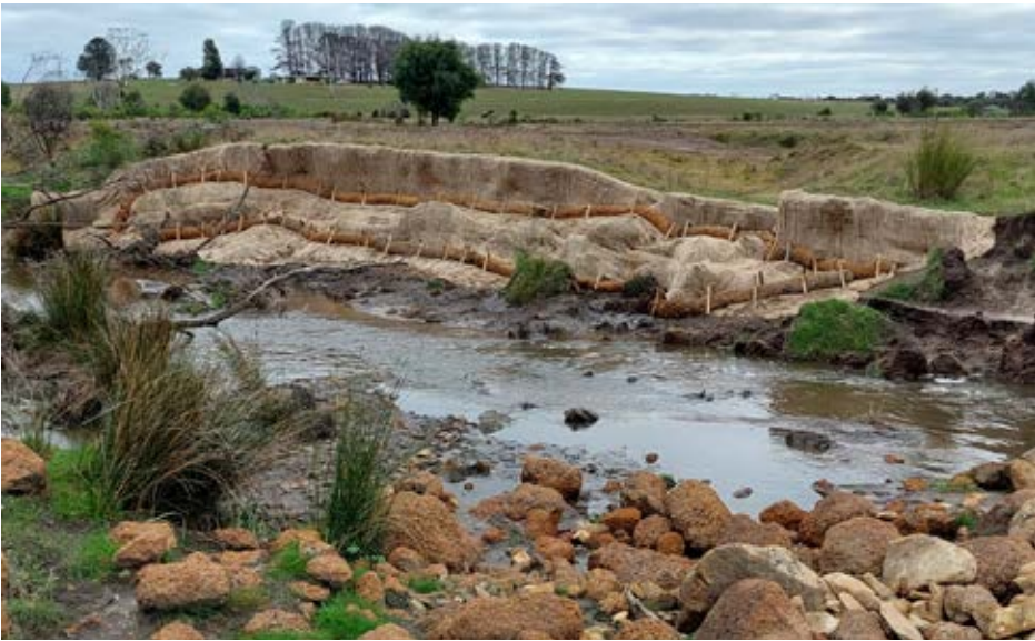
Image below: Erosion control structure installed to protect streambanks on the Stun'Sail Boom River.
