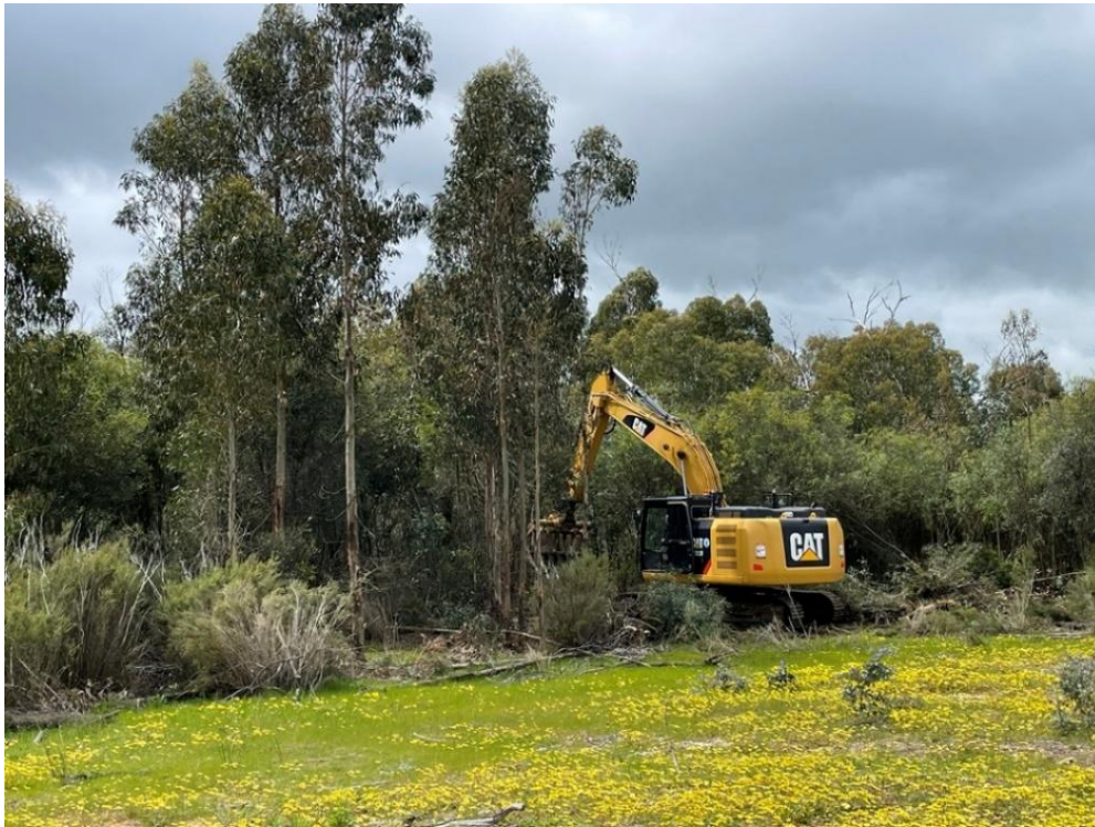
Figure 4. Stick Rake (Haby) - CAT Long Track Excavator with Stick Rake attachment operating at site H17.
