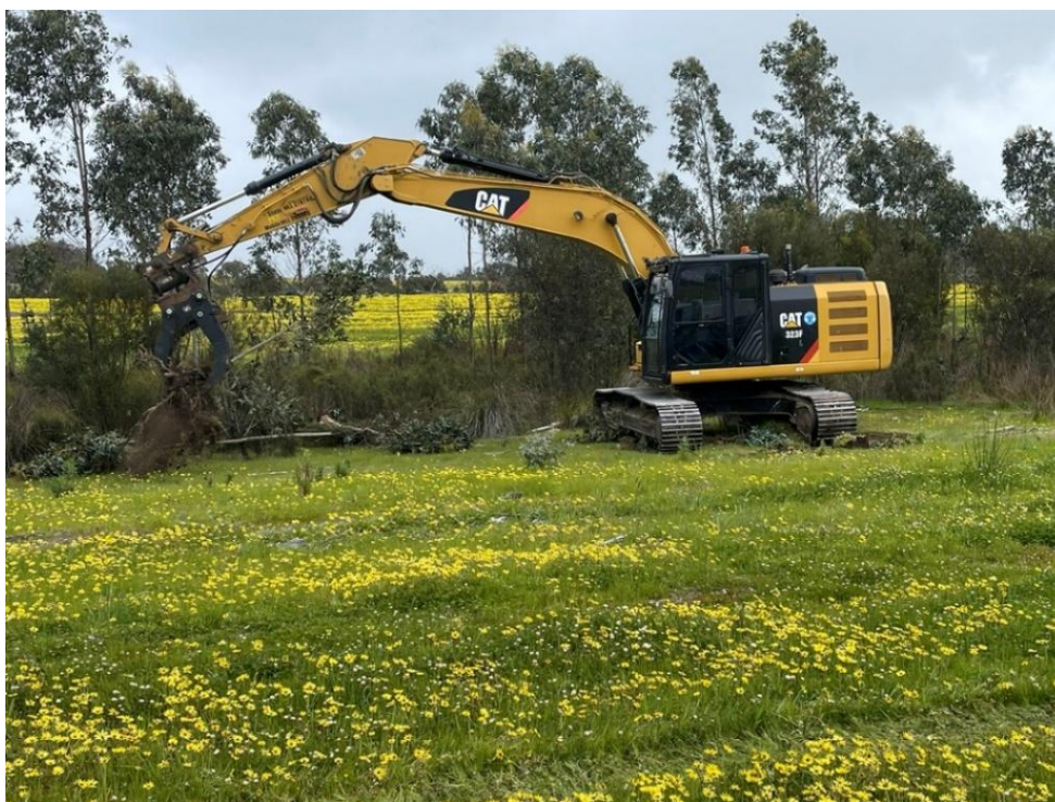
Figure 6. Grab (Haby) - CAT Long Track Excavator (162 Hp) (23 tonne) with Grab attachment operating at site H31c.
