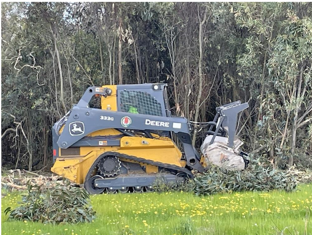
Figure 3. Forestry Mulcher (DEW) - John Deere 333G Compact Track Loader with FAE forestry mulching head operating at site L6.
