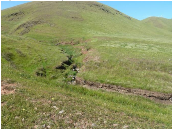
New Salt Creek – erosion caused by clearance of surrounding slopes
