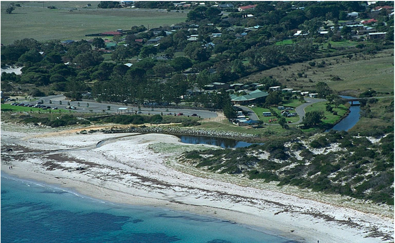
Normanville: the Bungala River Estuary, Normanville Dune, caravan park and carpark (Coast Protection Board, May 2003)
