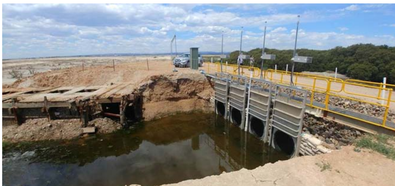
Figure 21. The tidal gate controlling inundation of XB8A. Photo: Chris Purnell
