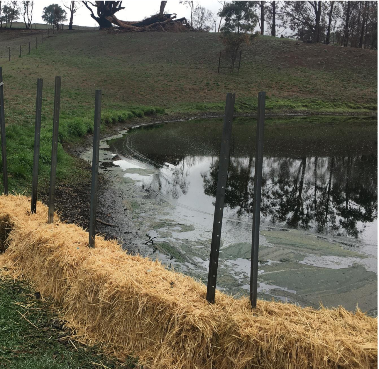
Farm dam at a Charleston property, with hay bales being used for sediment control
