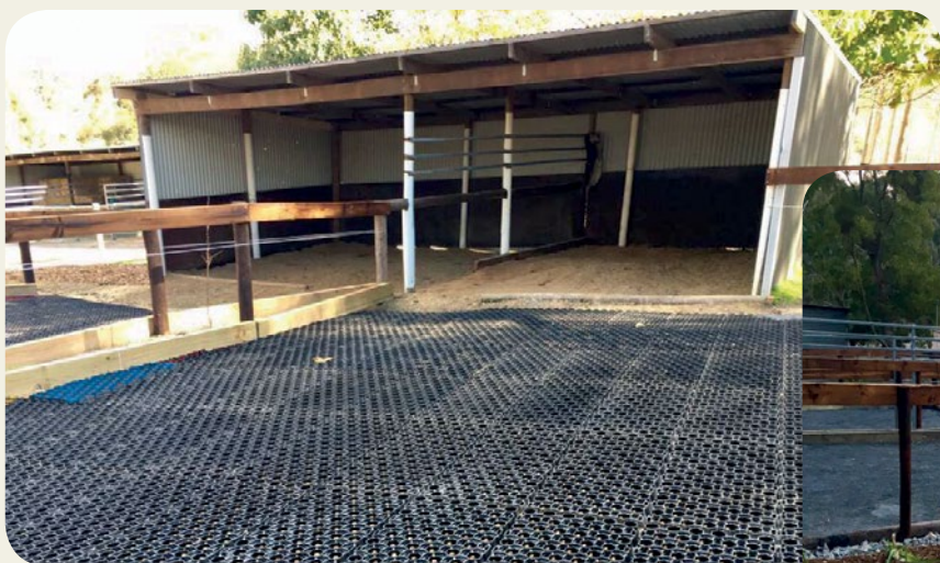
Geocell laid prior to surface overlay, reducing mud. Photos: Sue Brown
