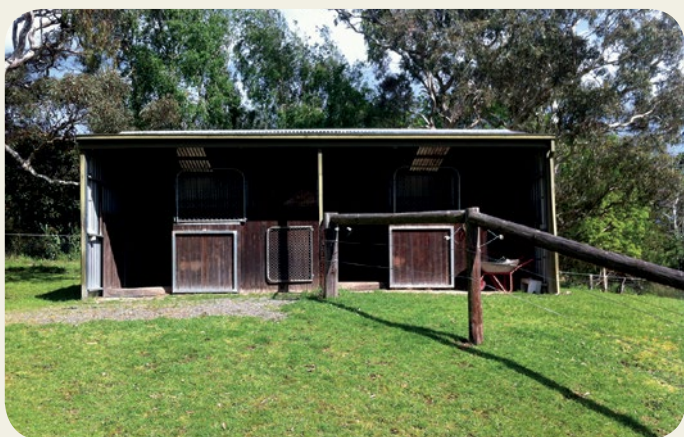
Stables sited on a slope: Kikuyu and coarse gravel help prevent erosion.
