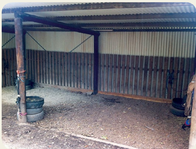
Horse shelter with timber lining.
