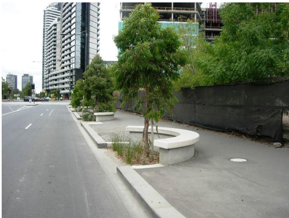
Figure 46: Batman Drive bioretention tree pits, Docklands Melbourne. By author.
