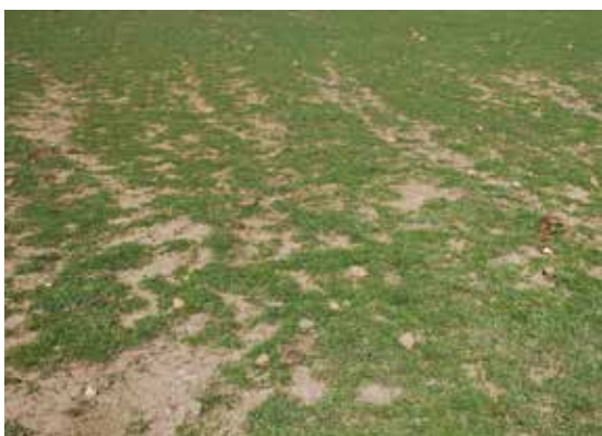
Figure 77. Erosion caused by insufficient ground cover
