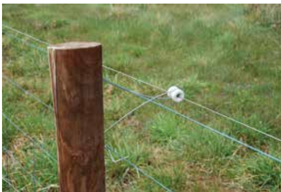
Figure 98. A single offset electric wire can be used to keep horses well away from ringlock fencing
