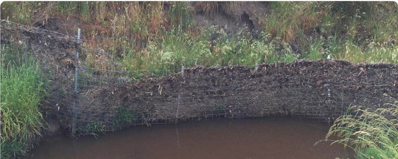
Alignment training - wire fencing
