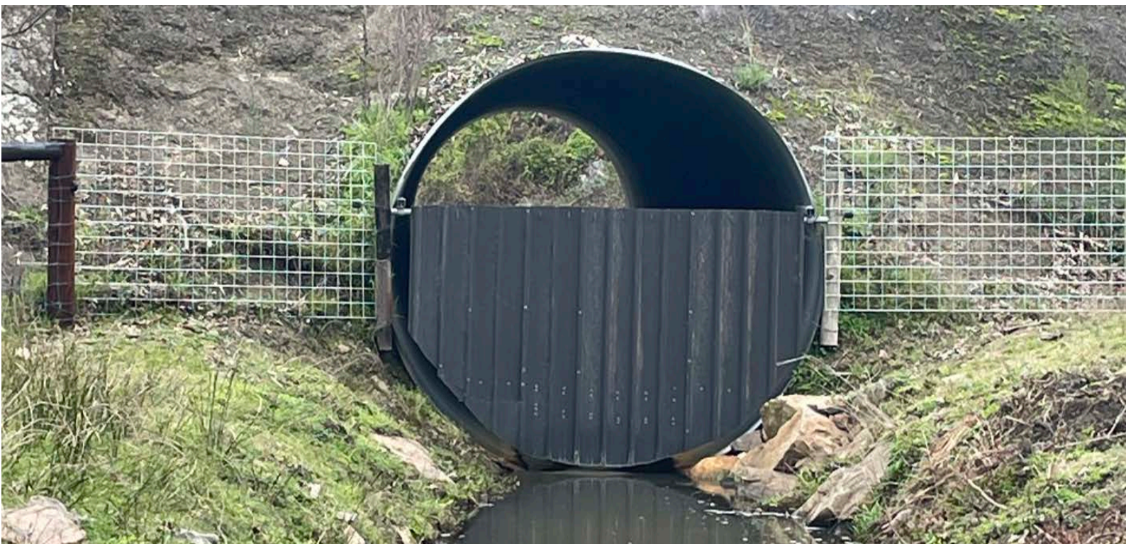
Flood gate fencing allowing for normal flow and fish passage
