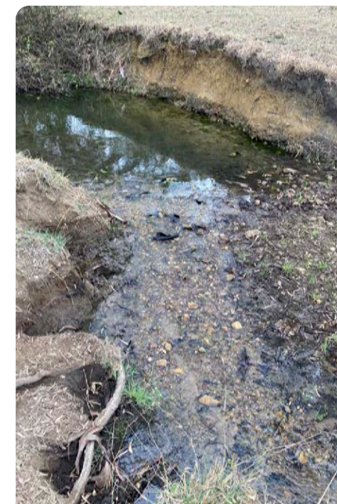
Bank slumping erosion
