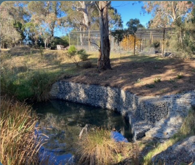
rock gabion basket for erosion issues threatening infrastructure
