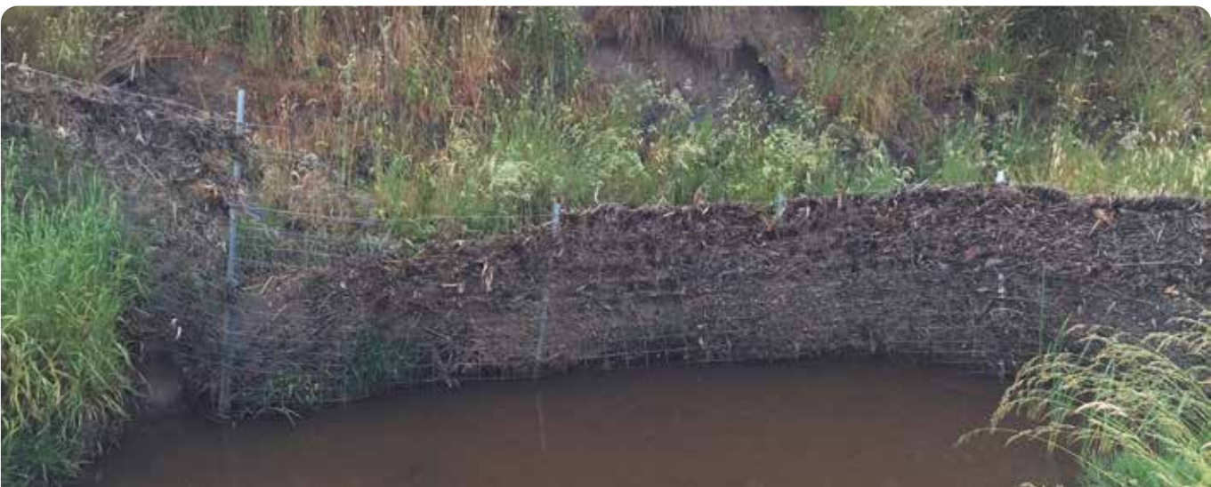
Alignment training - wire fencing
