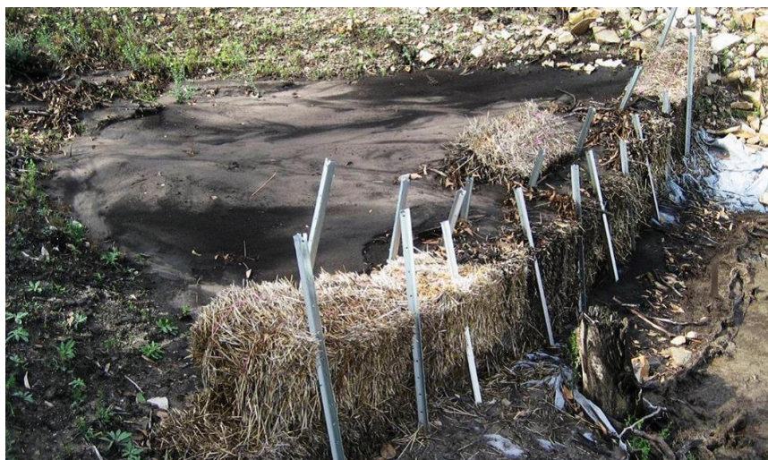
An example of sediment control using straw bales
