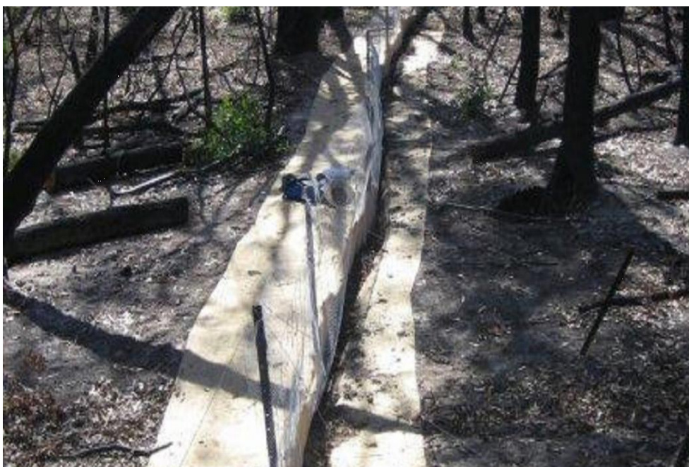
An example of sediment control using wire and hessian cloth.
