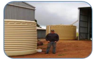
New tanks, key water storage infrastructure part of the new Water Plan
