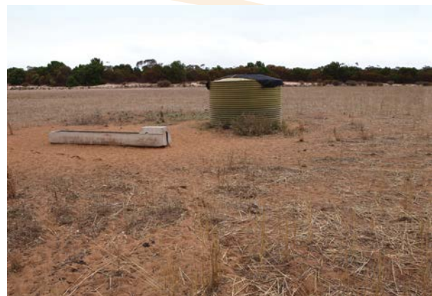
One of the holding tanks required for a new trough.
