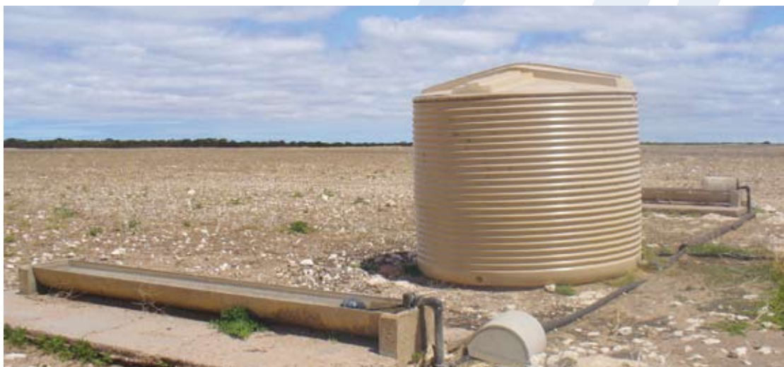
Concrete apron around trough to stop erosion.
