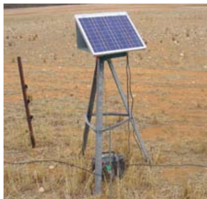
Solar energiser mounted on an old windmill stand.
