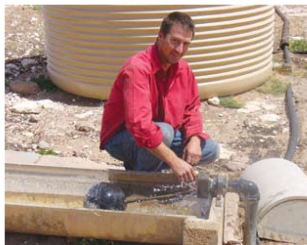
Richard Dutschke next to one of his troughs with a 50mm float valve.
