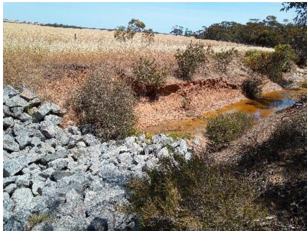
Placement of rock good size and placement, having previously been too small
