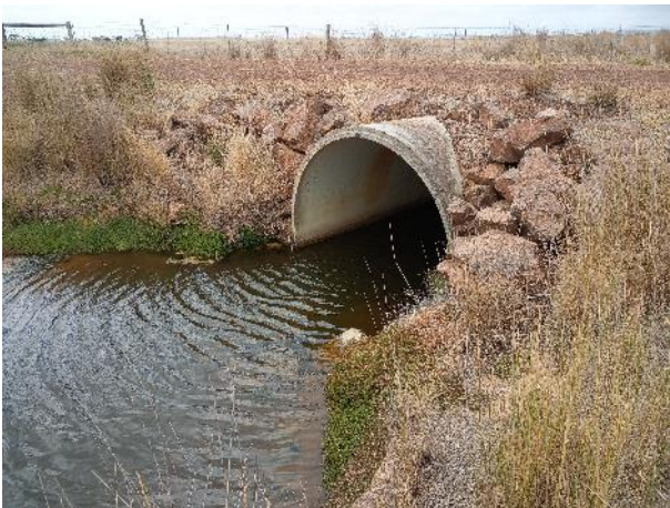
Culverts adequately sized, free flowing, and adequately protected from erosion
