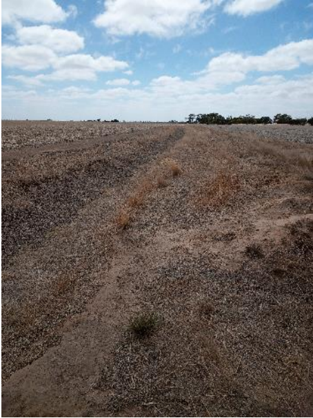
Trenches well designed and constructed:
