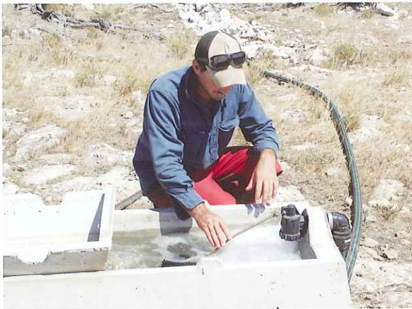
40mm float valve provides high flow rate.
