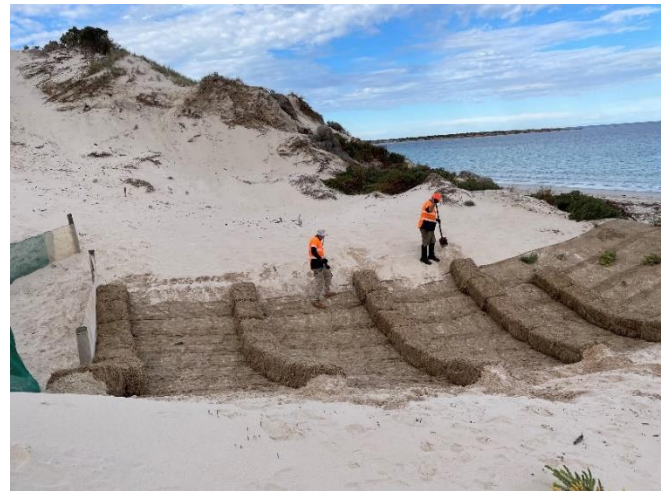
Photo 11: 'Coastal Management at Moonlight Bay' contractors rehabilitating a blowout area using a combination of hay bales, jute matting and erosion control fencing
