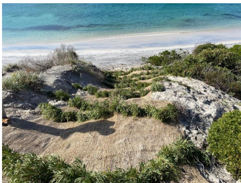
Photo 15: Jute matting and brush use in the rehabilitation works at Port Neill
