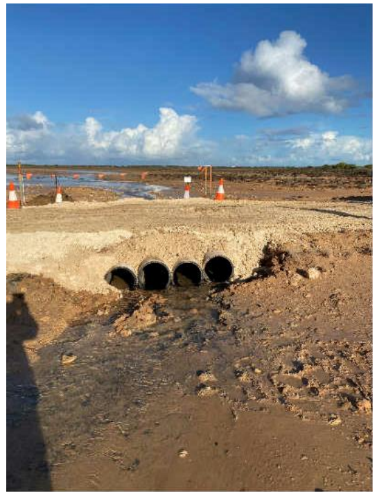
Photo 10: New culvert installed to restore tidal flows to supratidal samphire on the north side and supratidal and intertidal saltmarsh on the south side of Cowleys Road, Amo Bay
