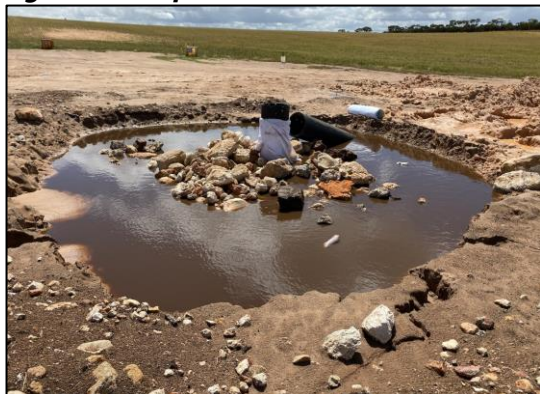
Figure 2. Sump under construction at Kimba 2.
