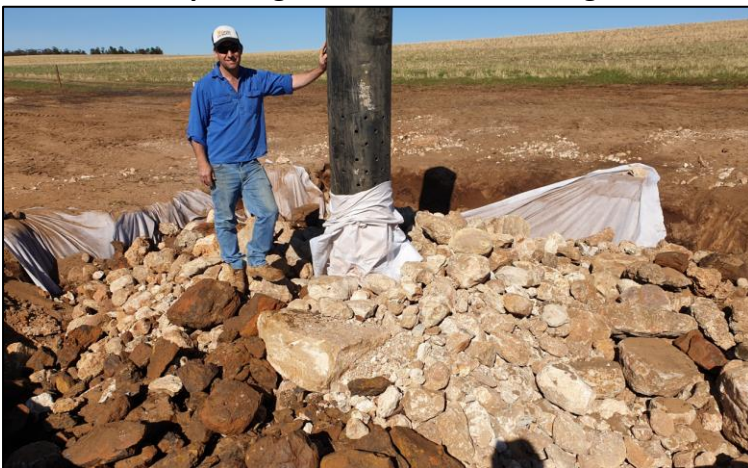
Photo 11. Sump area prior to final cloth and covering
