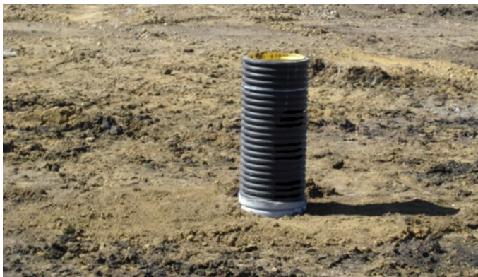
Proper well casing to access groundwater following a GAT rehabilitation.
