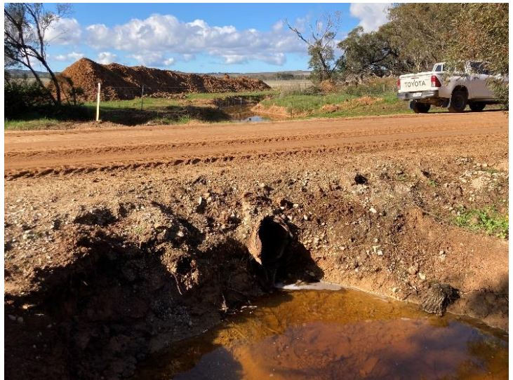
Photo 34: Cleanout of a road culvert and drain in the Lake Wangary Catchment
