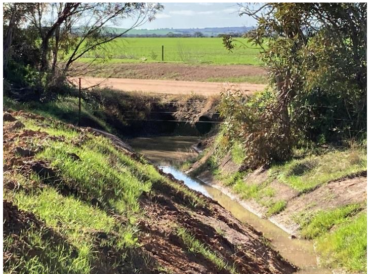
Photo 35: Cleanout of a road culvert in the Lake Wangary Catchment
