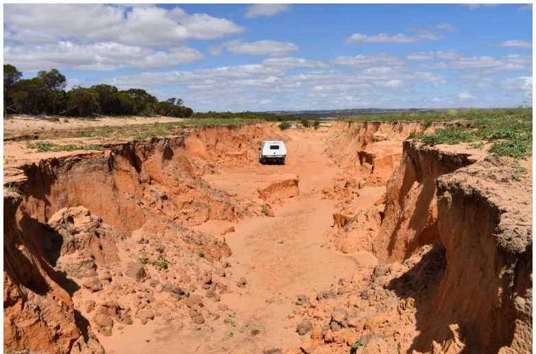
Photo 9: Extreme erosion gully on the northern side of Carippee Hill
