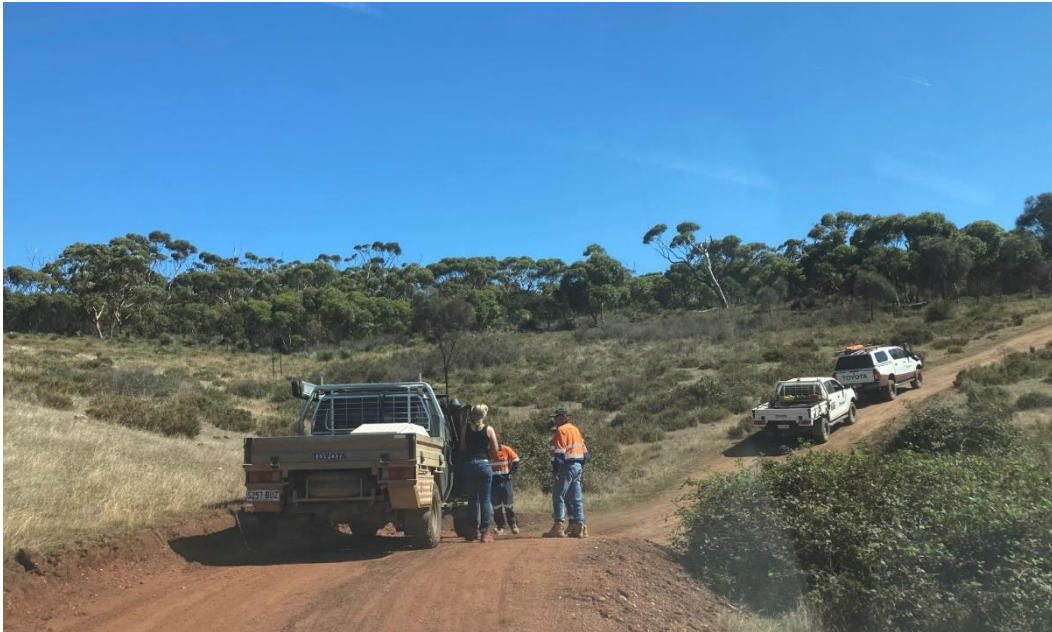
Photo 3: Site visit with Downer to look at progress of access tracks and creek crossings for ElectraNet High Voltage Transmission Line construction
