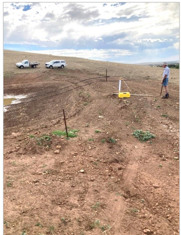
Photo 2: Completion of works inspection and survey on new dam with an insufficient spillway capacity
