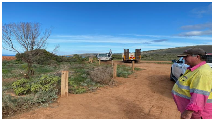
Photo 23: Post and chain vegetation barriers installed to delineate camping areas and protect vegetation from vehicle damage.
