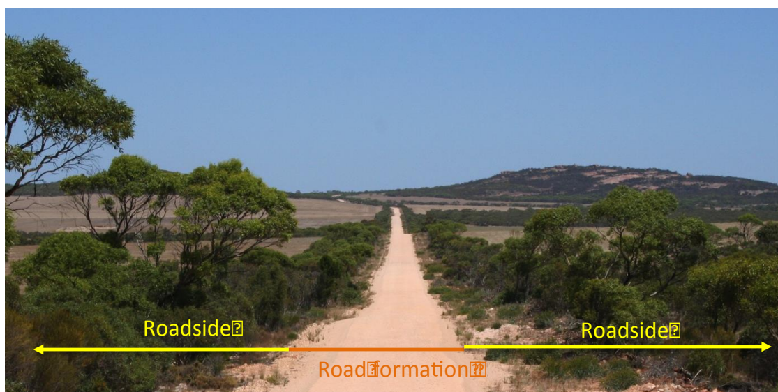
Figure 2: Road reserve showing the road formation and the roadsides.
