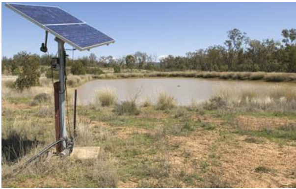
A farm dam on Eyre Peninsula equipped with a solar-powered water pump.
