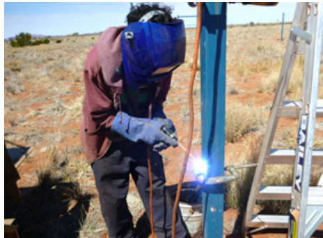
Roland Baker welding
