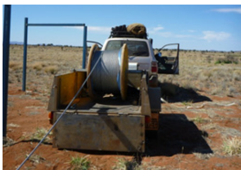
Cable drum set up on trailer
