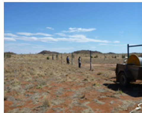
Welding cable guides to posts and running out the wire
