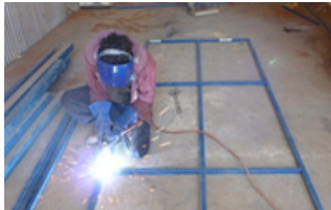
Welding gates at Kampi Community shed
