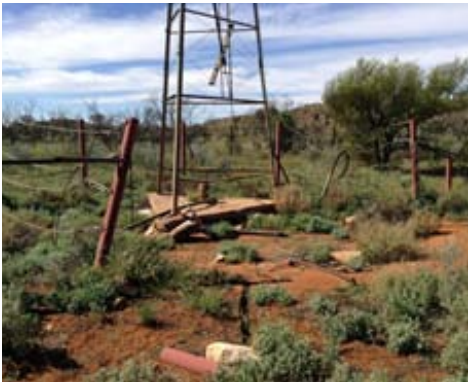
Damaged fence at Angatja Well
