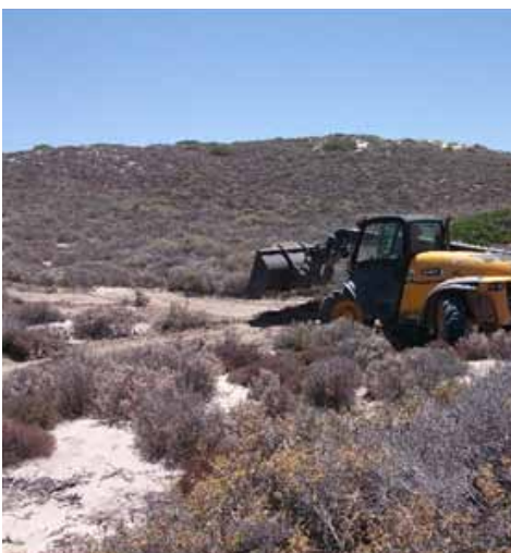
Clearing the bin area and driveway access was undertaken using heavy equipment to provide a flat surface
