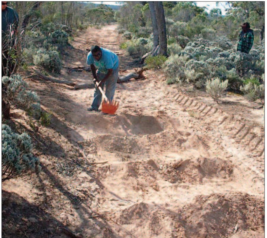
YLM Ranger, Mark Young, preparing a track with water runoff for direct seeding.
