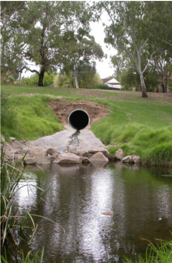
stormwater outlet
