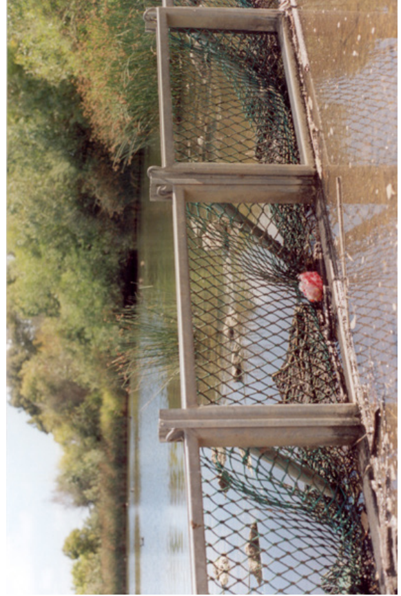
litter trap (trash rack)
