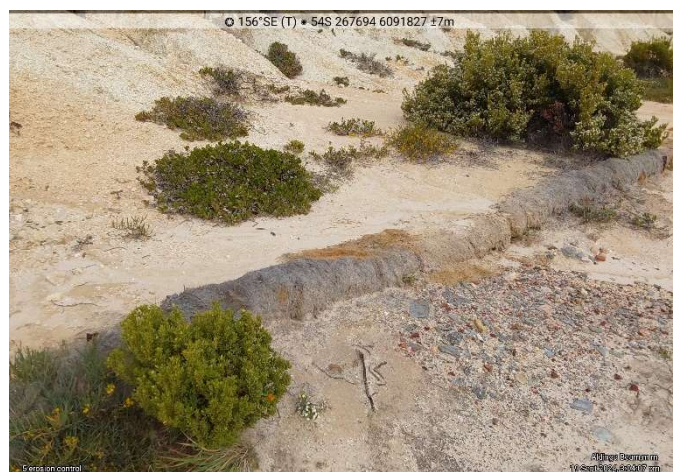
Figure 4.7 (above right) Various erosion control techniques have been trialled at this location, with coir logs (pictured) being successful at trapping sediments and facilitating recovery of the toe of the slope.
