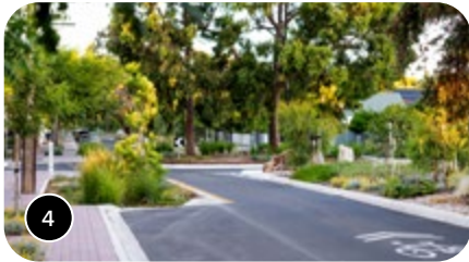
Retrofit for corridor planting, St Peters Streetscape. Source: Sweet Lime, photography by Duncan McKenzie
