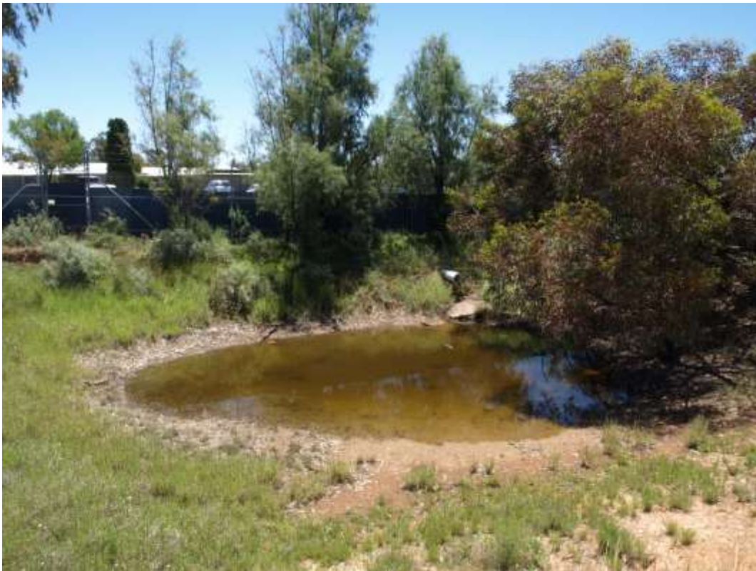
Photo 2 Storm water retention basin with planted trees.
