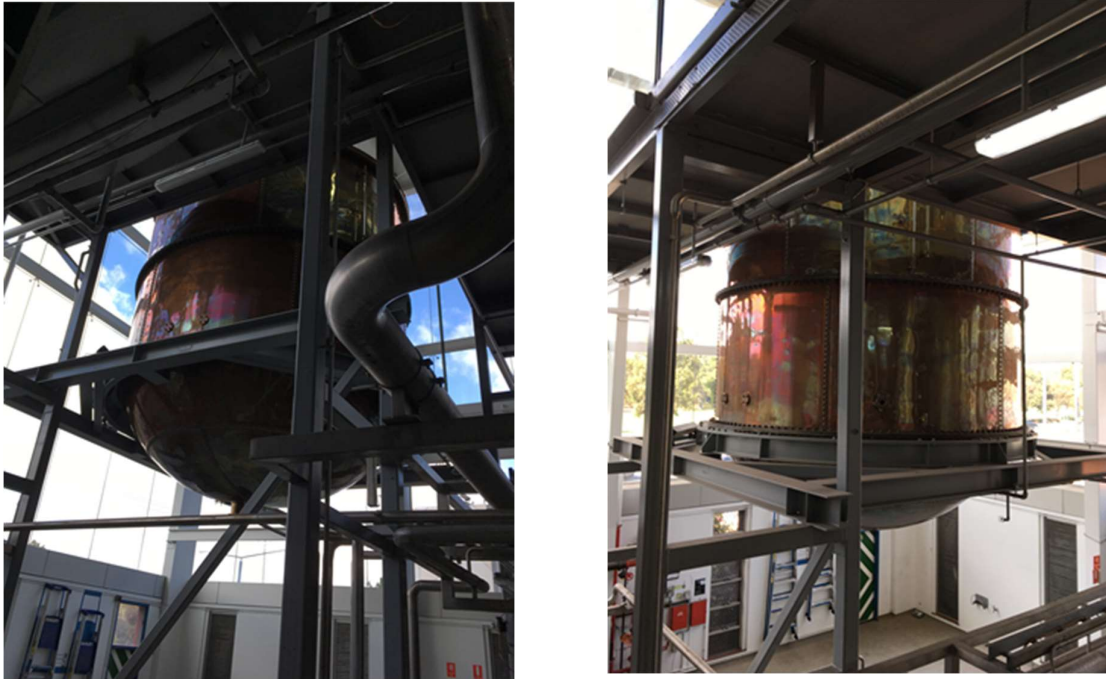
Copper kettle, showing riveting and rounded base. Source: DEW Files 24 March 2021.
