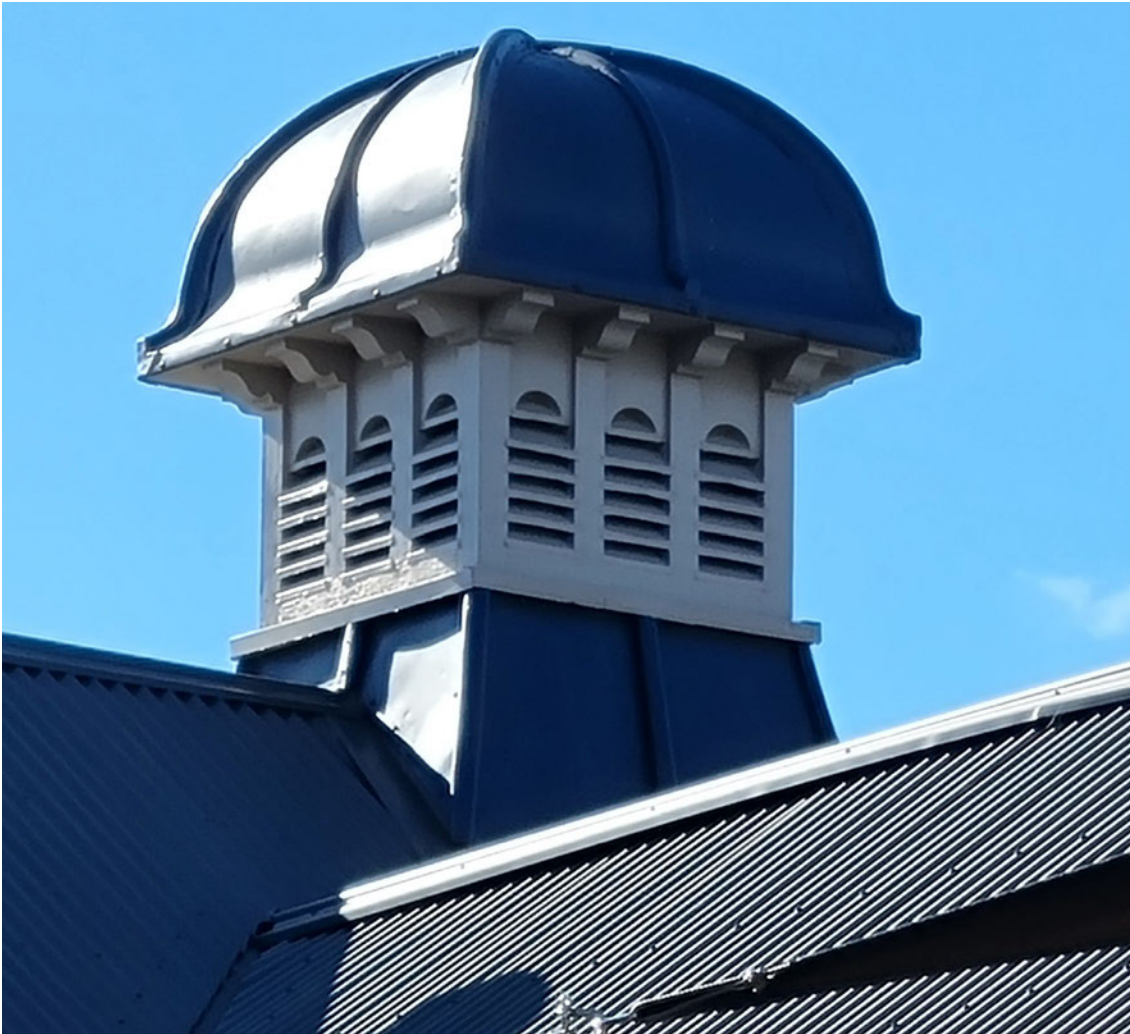
Figure 23: Rosary Hall, wooden square bell ventilation 'cupola' dome, 13 April 2022 (photo taken by Applicant)
