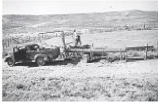
Pumping water from the tank c 1960's
