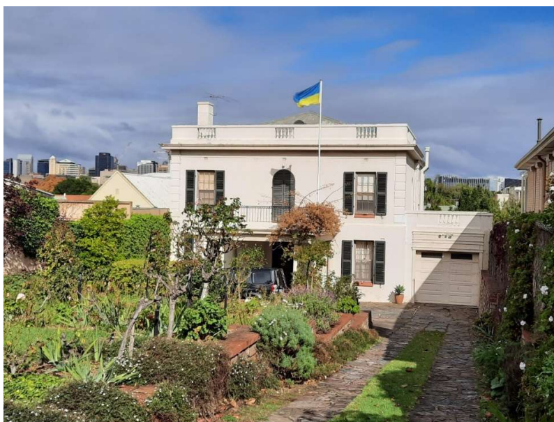
Photo: 92 Brougham Place, North Adelaide. Source: DEW files
