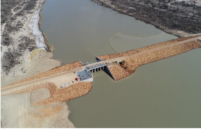
Pike River regulator and Fishway Image: Dan Haines SA Water
