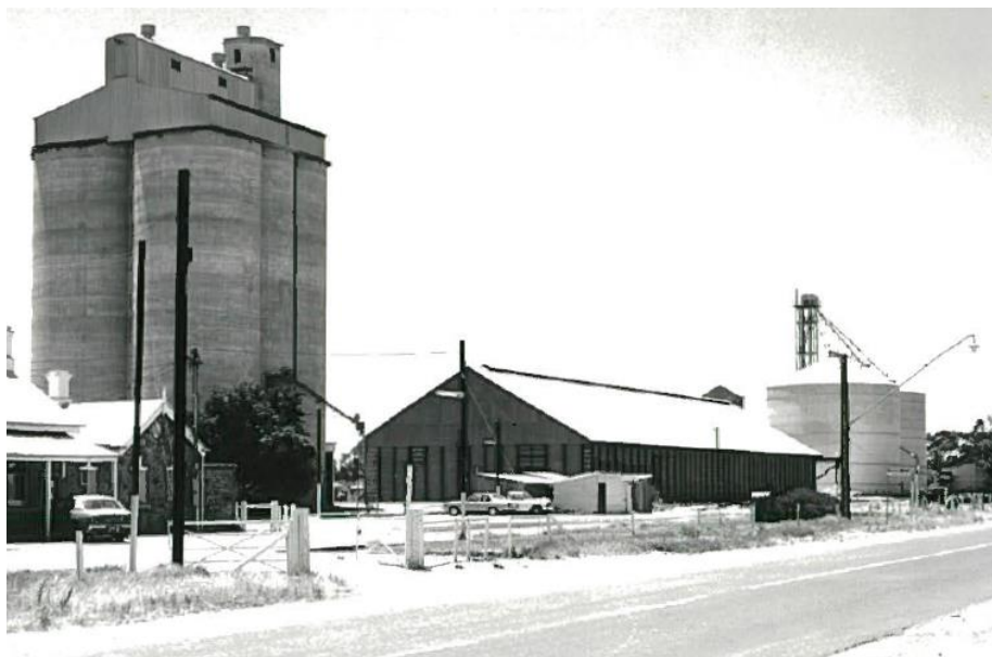
Railway Station Complex and Silos at Balaklava (SHP 12942). All three silos, cylindrical concrete vertical (on left), steel horizontal (centre), and cylindrical steel vertical (on right) were built by SACBH. The horizontal steel 'shed-style' silo was the first silo erected on the site in 1956.
