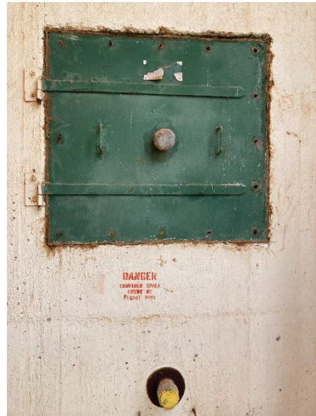
Detail of direct access door to the inside of one of the silo cells.
