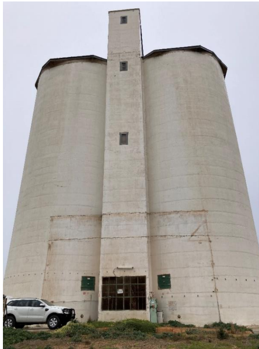
South-east side of the Nantawarra Silo. Note the rectangular outline at the base marking where the hopper enclosure once was. The ground in front is where the receival hopper has been filled in.
