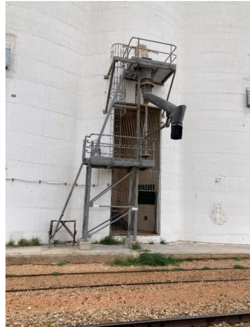
Detail of spout that feeds grain from the silo into the railway cars for transport.
