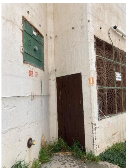
Entry door at the base of the elevator. The door on the left provides direct access to the inside of the silo cell.
