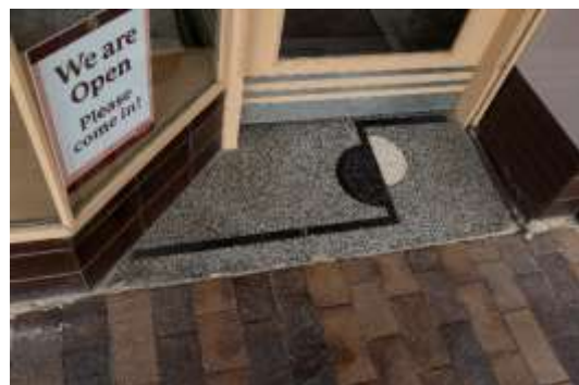
Terrazzo re-entrant floor to Shop 1
