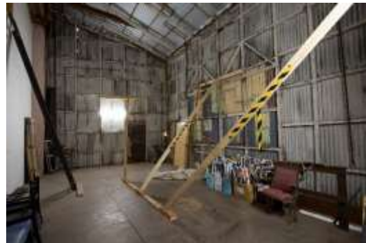
Interior stage house
