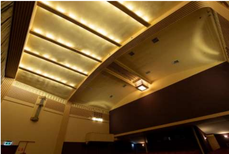
Downstairs auditorium ceiling
