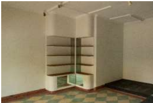
Terrazzo and corner display case in Shop 2
