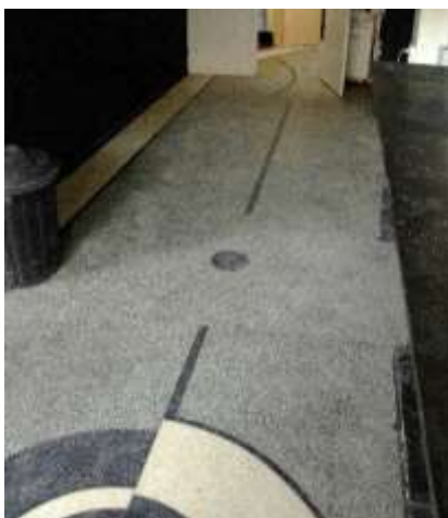
Side exit terrazzo floor
